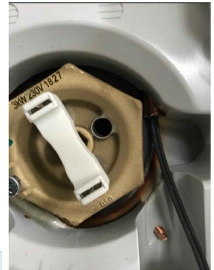
For Daikin 300ltr tank fix the tank thermistor in the opening like image
